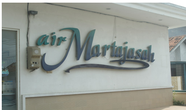
Figure 15. Building of Martajasah water management
